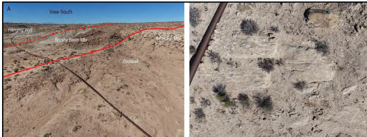
Figure S5C- 4. Left: Perspective view looking south where the red trace is the fault crossed by the pipeline. Brann Johnson is at the fault contact crossed by the pipeline for scale. Right: Drone image looking down at a zone of deformation bands in the Salt Wash sandstone at the location of Brann Johnson in the left figure. The pipeline is in the upper left. Drone photos by R. Cole.
